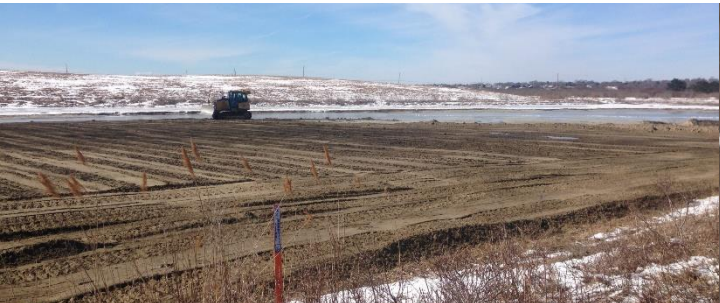
Thin layer deposition of sand from upland source on low marsh area
