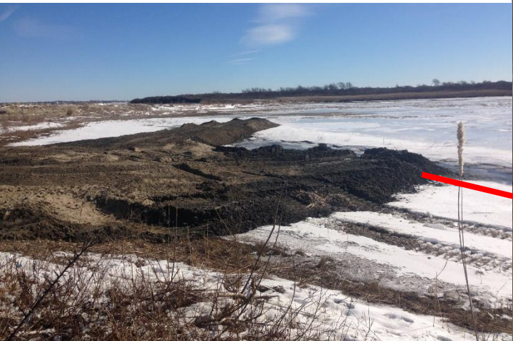
Thin layer deposition of sand from upland source on low marsh area
